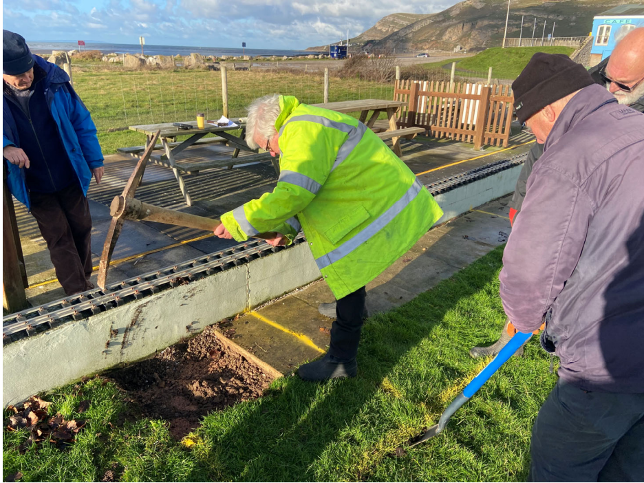
Start of the project with Tony in charge of the pick.
